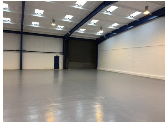
*typical interior post landlord works
